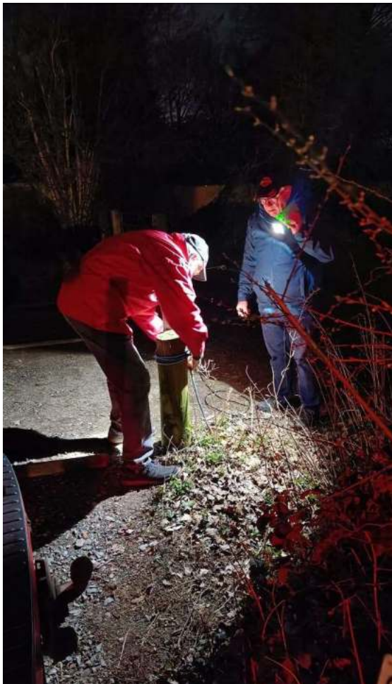
Dave G8FMC & Roger 2E0TGU ( Holding the torch was an important job! ) attaching antenna wire to 49:1 transformer
