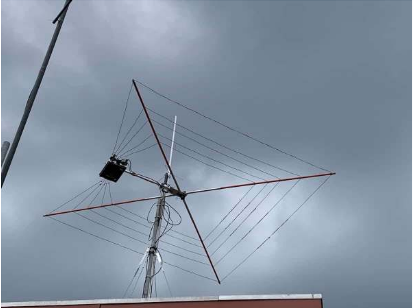
The CG-3000 remote tune at feedpoint of the Cobweb antenna.
