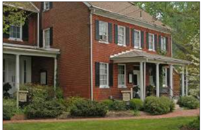
Elkeridge Furnace Inn, Furnace Avenue
